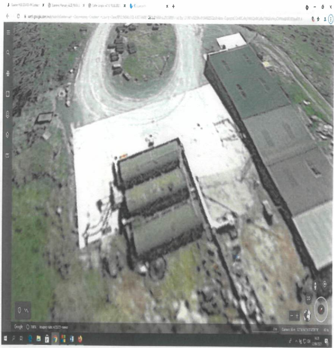
Google Maps 2021 Missing Bunding Walls
